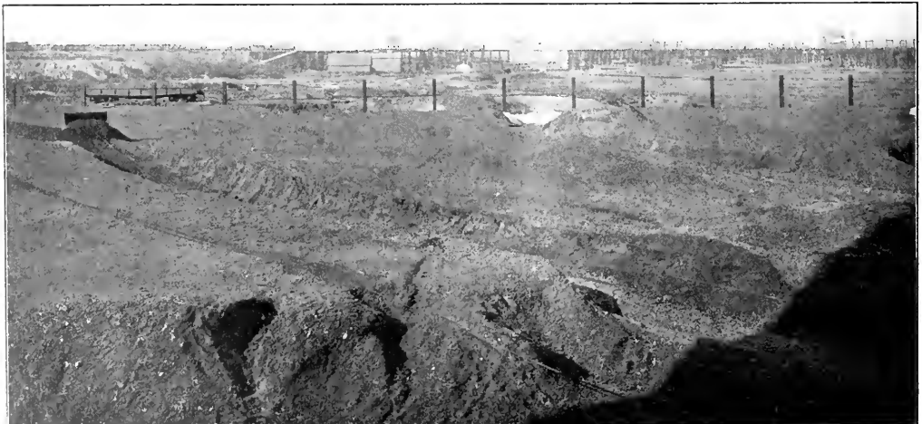
FIG. 1 STORAGE YARD IN WHICH 11,000 TONS OF COAL ARE HANDLED YEARLY
